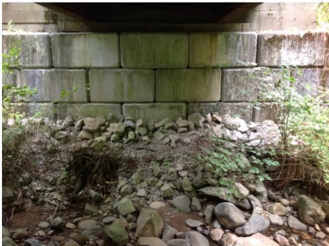
Right Bank Abutment when facing downstream
