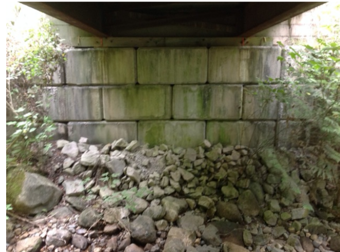
Left Bank Abutment when facing downstream
