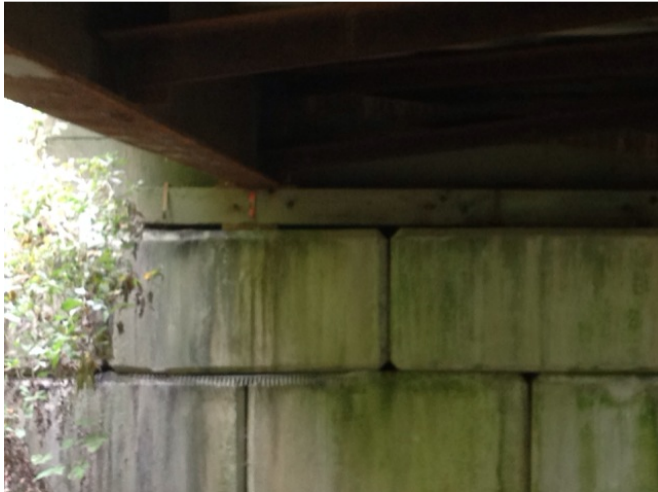
left upstream bearing shimmed level
